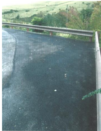
Bettws parish hall car park, after stabilising + resurfacing . 2021
