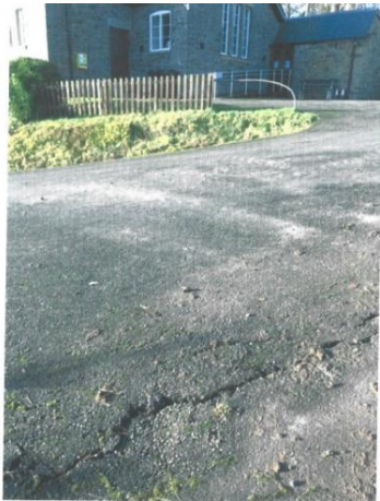
Bettws parish hall car park - before
